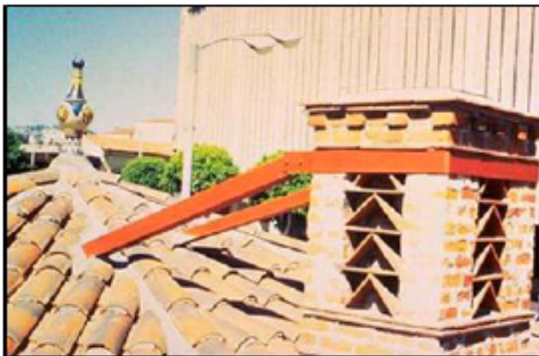
Figure 32 Chimney Restraint
