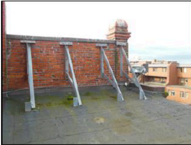
Figure 31 Parapet restraint.
