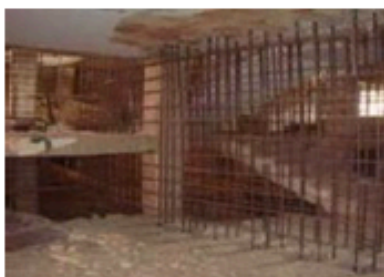
Figure 40 Replacing existing masonry walls with reinforced concrete walls.
