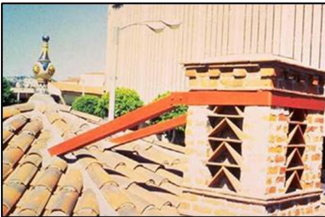
Figure 32 Chimney Restraint
