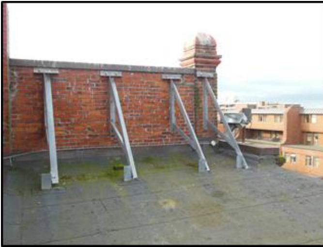
Figure 31 Parapet restraint.
