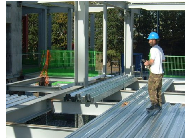
steel-concrete composite floor systems
