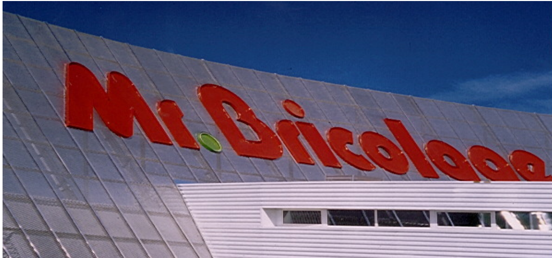
Centre commercial – la Roche/Yon (France)
