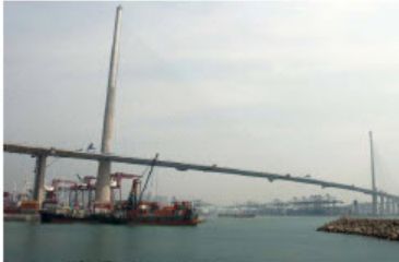
Figure 1: General view of Stonecutters Bridge
