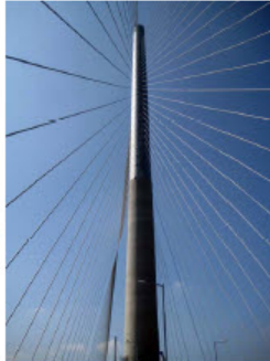
Figure 2: Mono tower and stay cables
