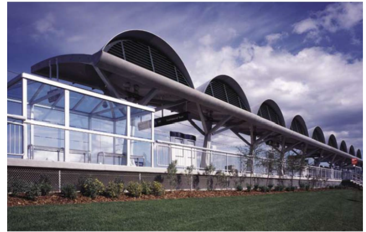
UHPC Roof elements: Shawnessy station at Calgary, Canada
