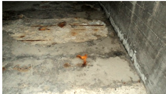
Performance of earlier repairs
