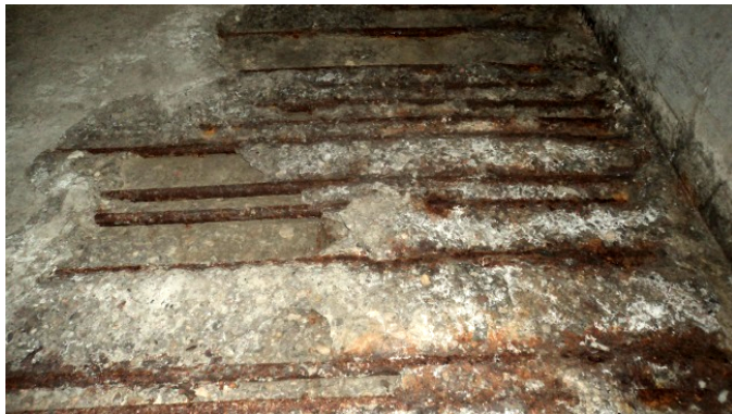
Damage in ventilation tubes, 2015
